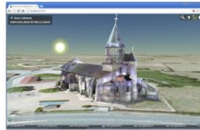
Point cloud of the Church of St Marie at Chappes, France.
